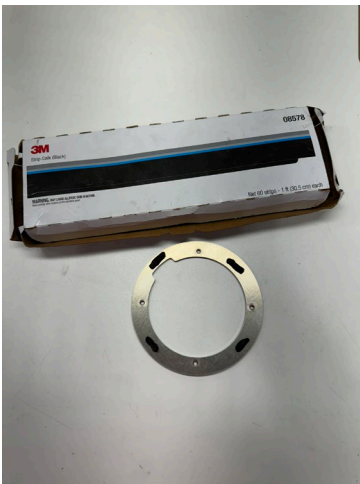
Step 4: Apply strip caulk to backer plate. (Prevents face of plate from butting against metal roof. Strip caulk face down towards headliner)
